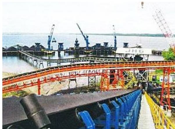
The coalmine inloading system conveyor system in Balikpapan, Indonesia, constructed by Maemode.
